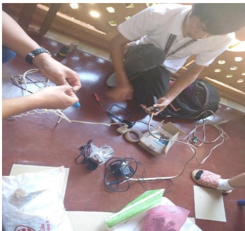
Installation of Wirings and System for Humidification
