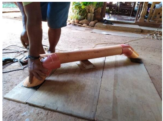
Installation of Piping for Air Distribution
